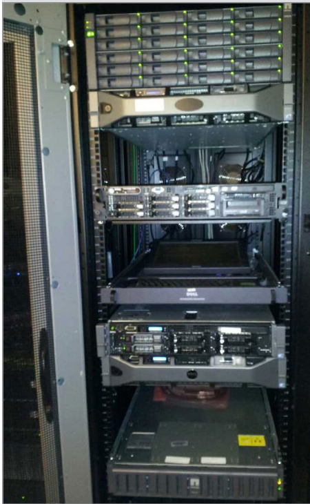
Figure 24. Level 4 Rack and Servers Located in an Energy Operations Center or Facility Operations Center
