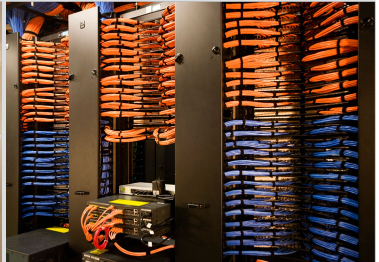
Figure 23. Level 5 Racks and Servers Located in a Facility Operations Center/Security Operations Center/Energy Operations Center
