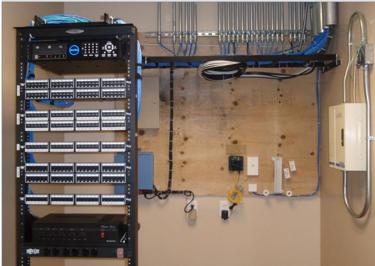
Figure 22. Level 5 Demarcation Point or Main Point of Presence Where the External IS Meets the Internal Building OT Interface
